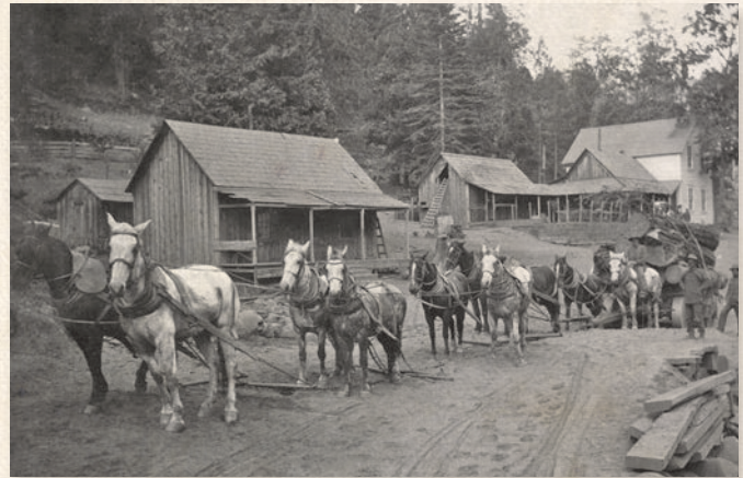
A Mule Team Pulling a Timber Cart
