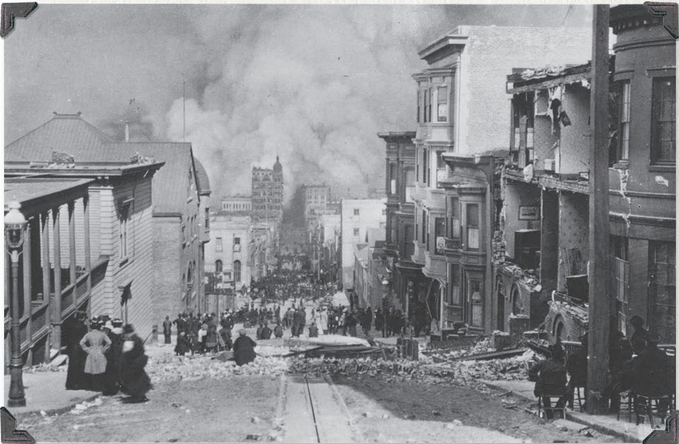
San Francisco 1906 Earthquake
